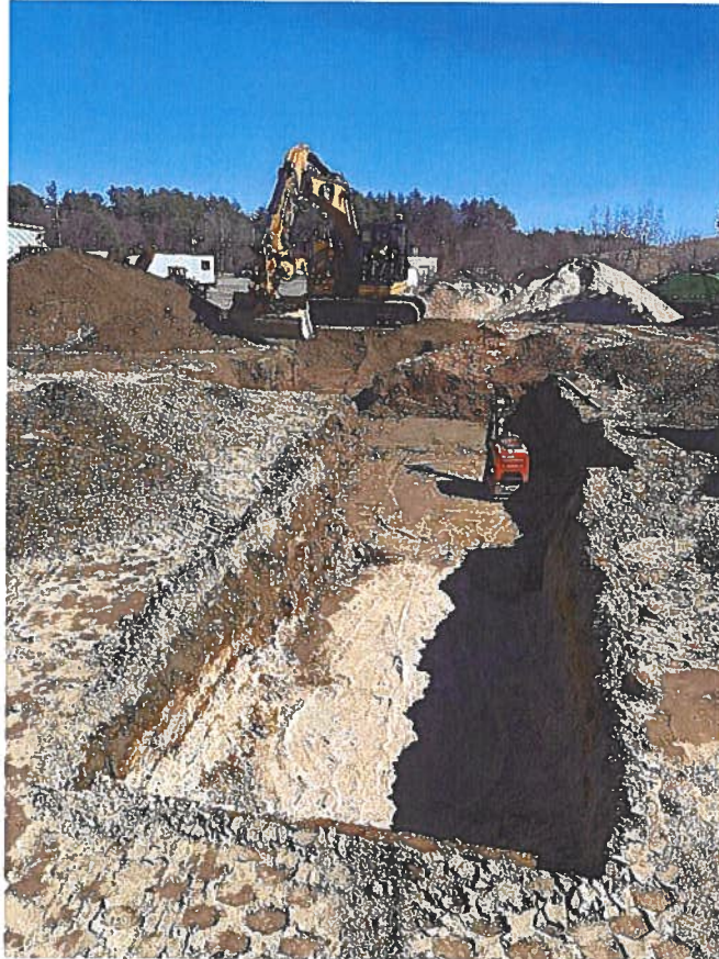
Preparation of subgrade for foundations – 3/22/22
