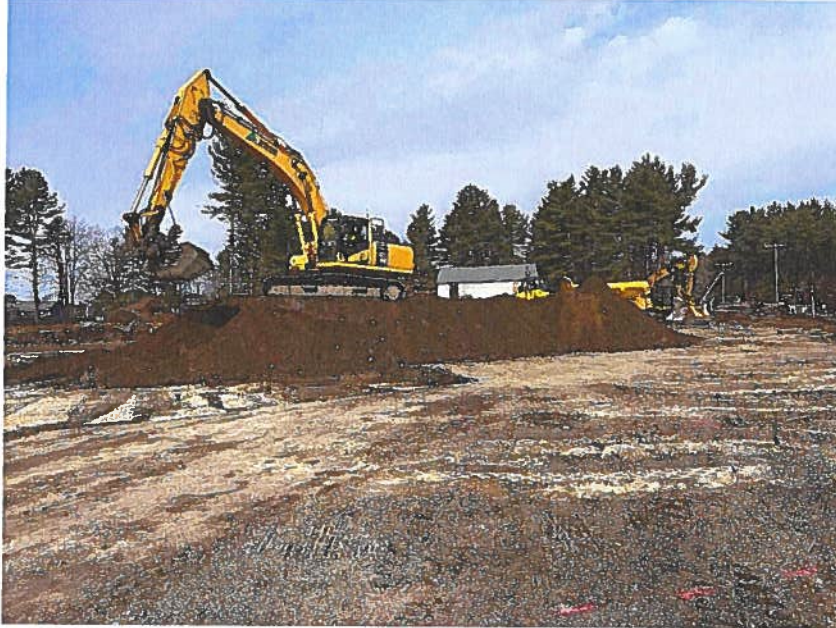
Excavation of unsuitable material (cont'd) – 3/15/22
